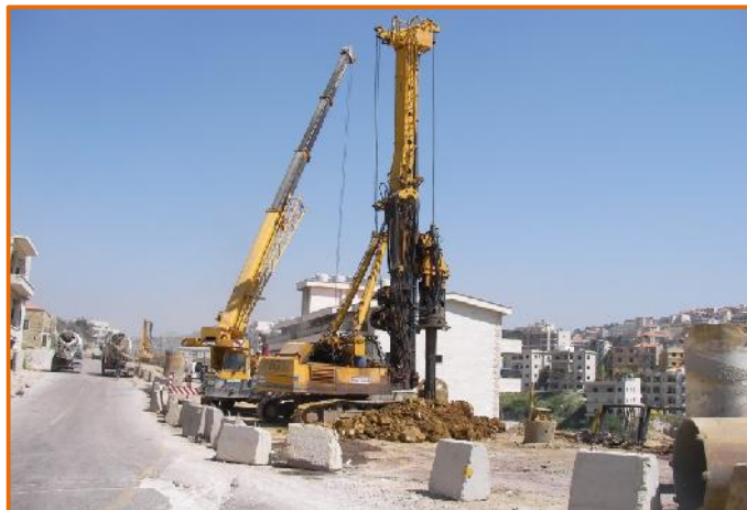
Piling operations underway in Bhamdoun
