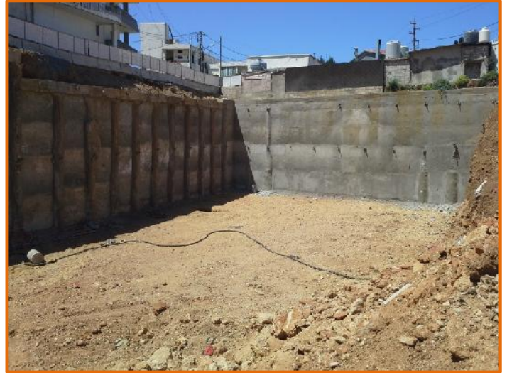
View of shoring from excavation level
