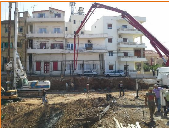
Pile concreting operation underway
