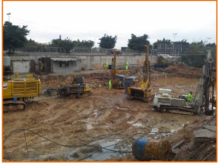
Grouting Operations under way
