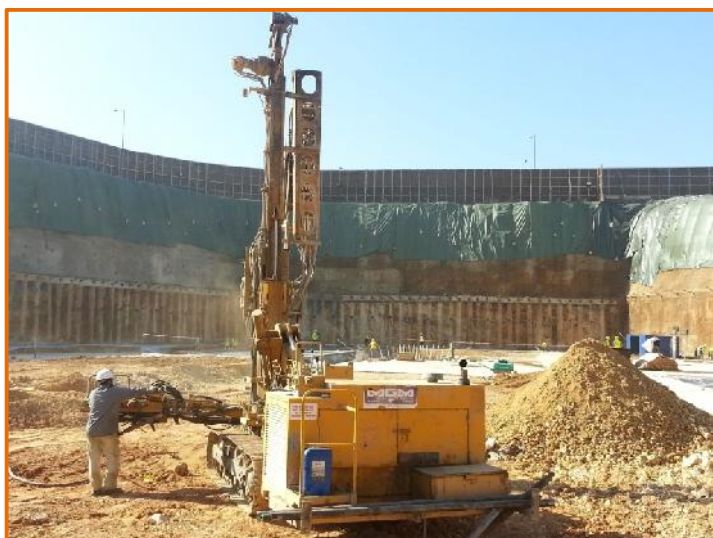
Cavity probing works underway
