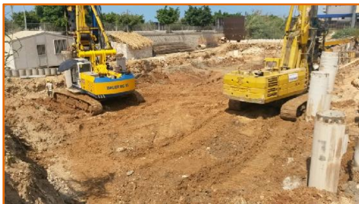
Piling Operations under way
