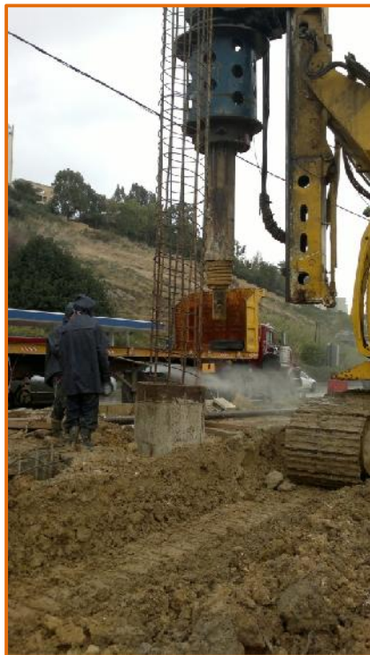
Piling process underway
