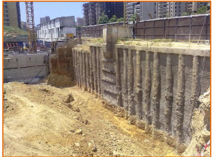
General View of Excavated Site Area
