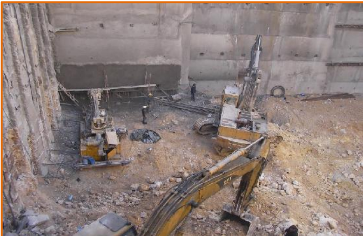
Excavation process underway
