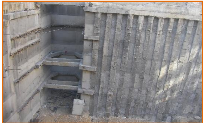
General View of Excavated Site Area
