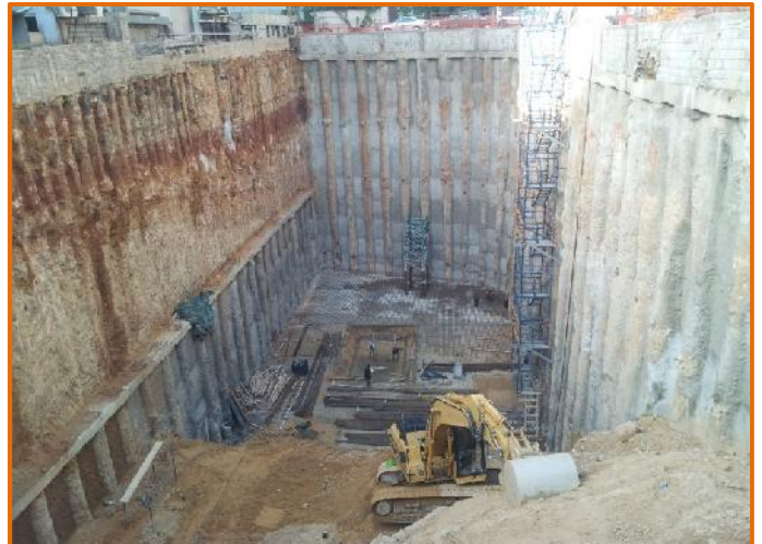
General View of Excavated Site Area
