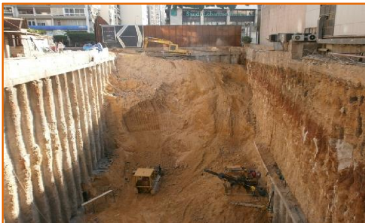
Excavation process underway
