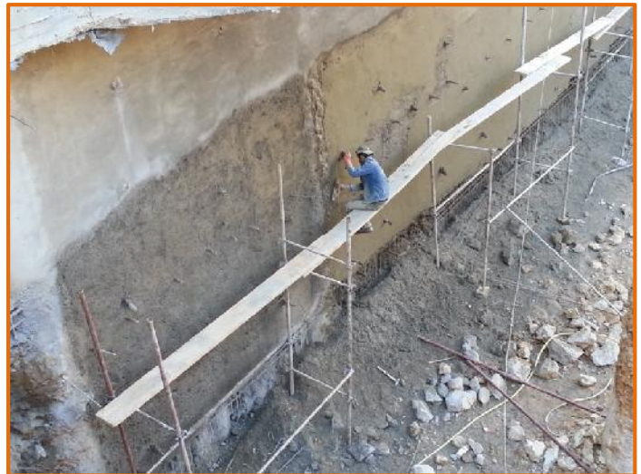
Smoothing of shotcrete facing
