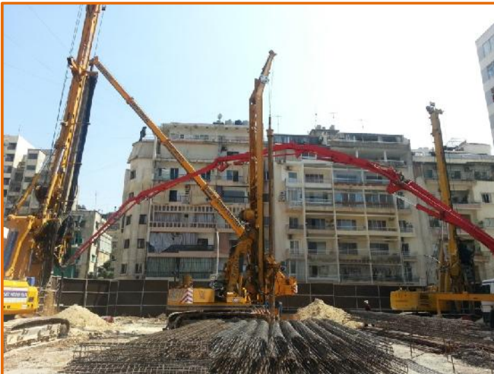
Piling Operations under way
