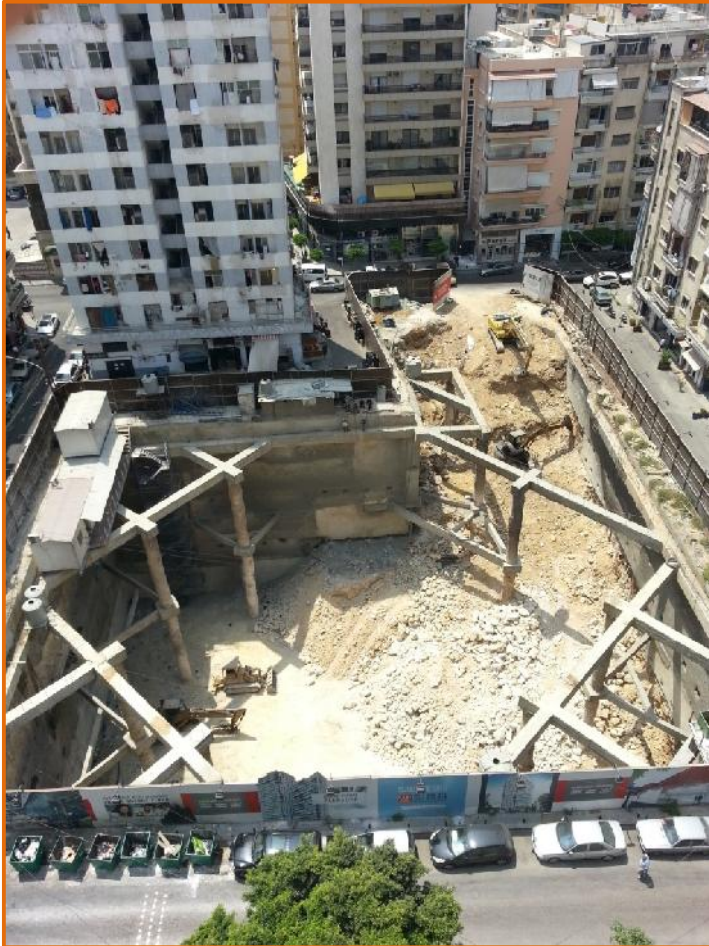
View of site with excavation works underway
