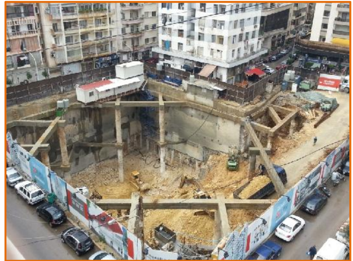
General View of Excavated Site Area
