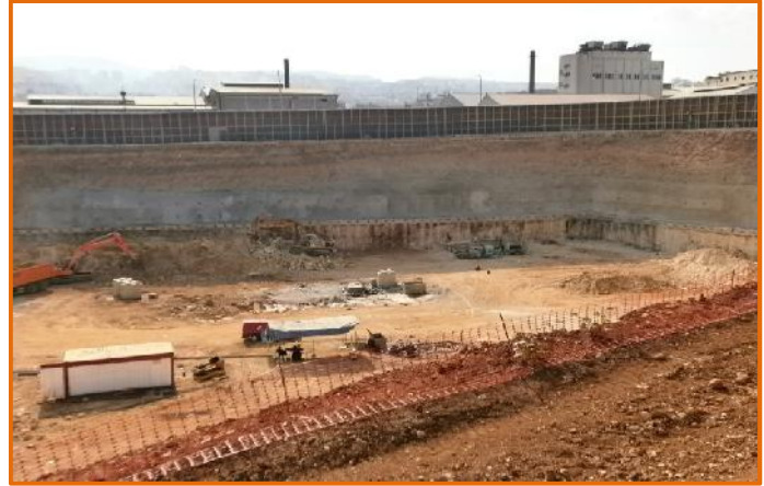
General View of Site Area
