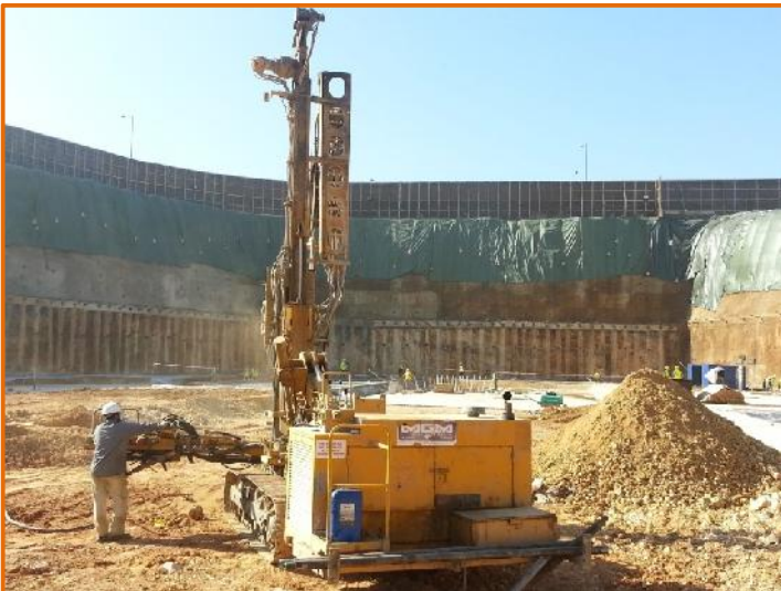
Cavity probing works underway
