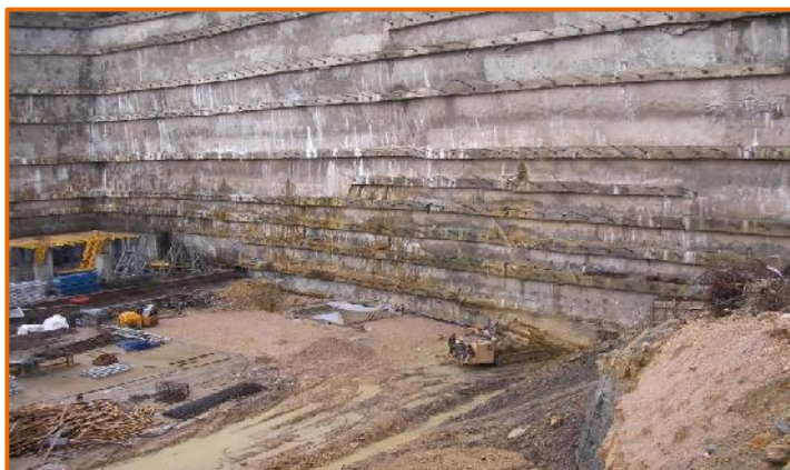
Anchor drilling operations underway
