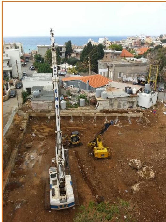
CMV Machine operating on site
