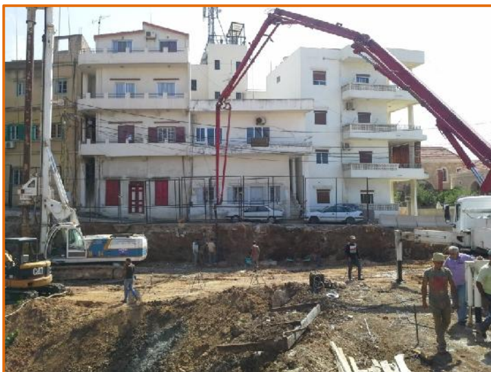
Pile concreting operation underway
