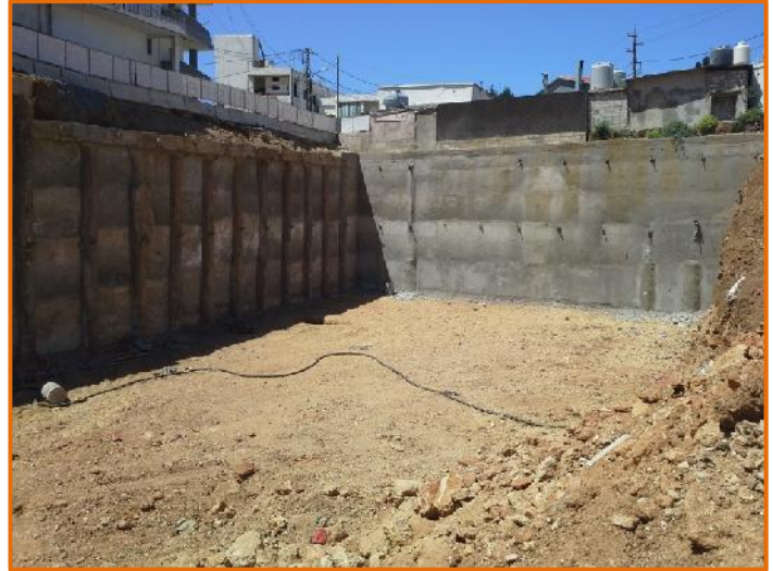
View of shoring from excavation level
