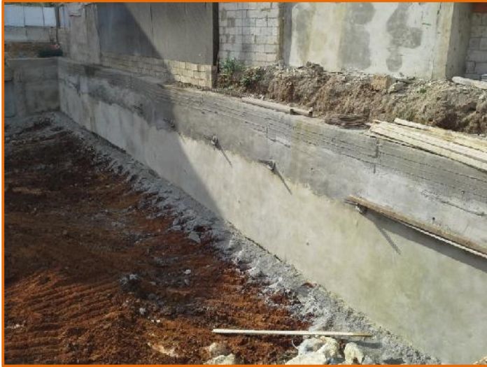
Shotcrete smooth finish
