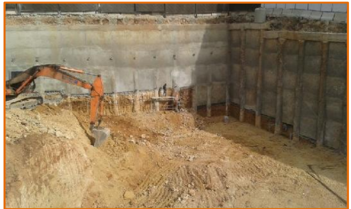
General View of Site Area
