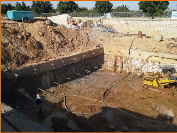
Shotcrete Operations under way
