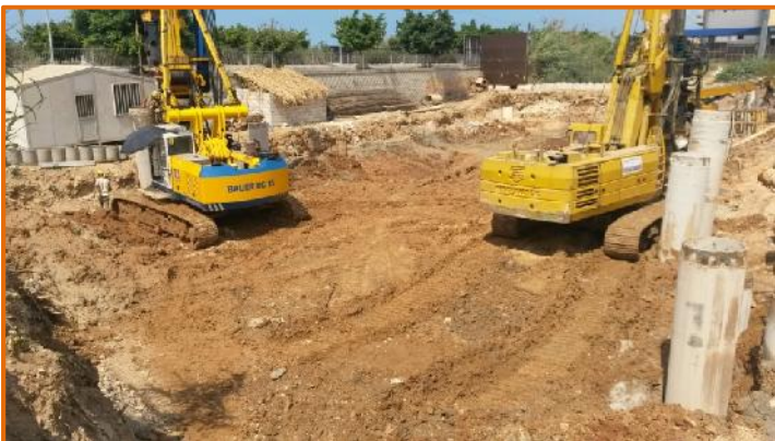
Piling Operations under way
