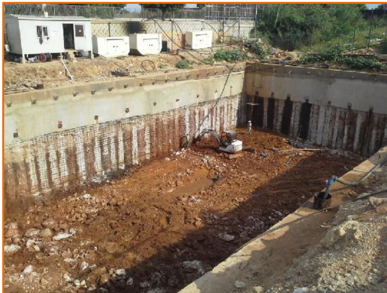
Excavation and shotcrete works
