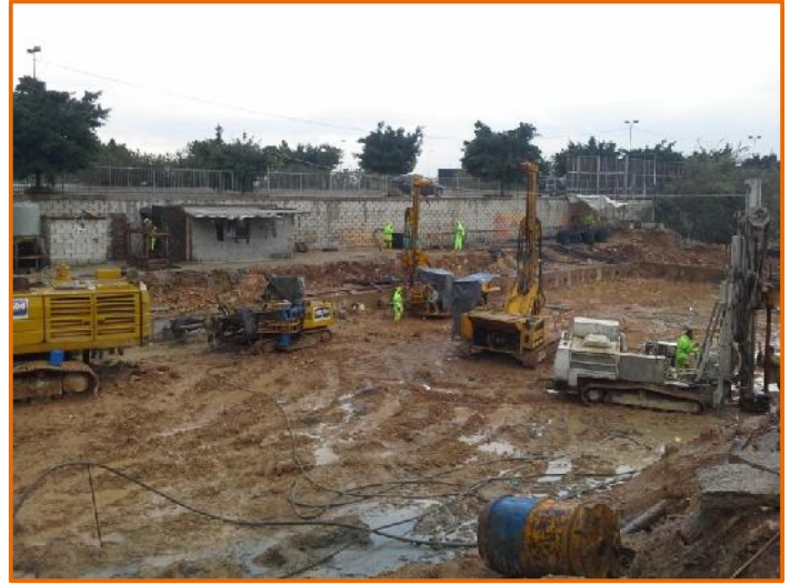
Grouting Operations under way
